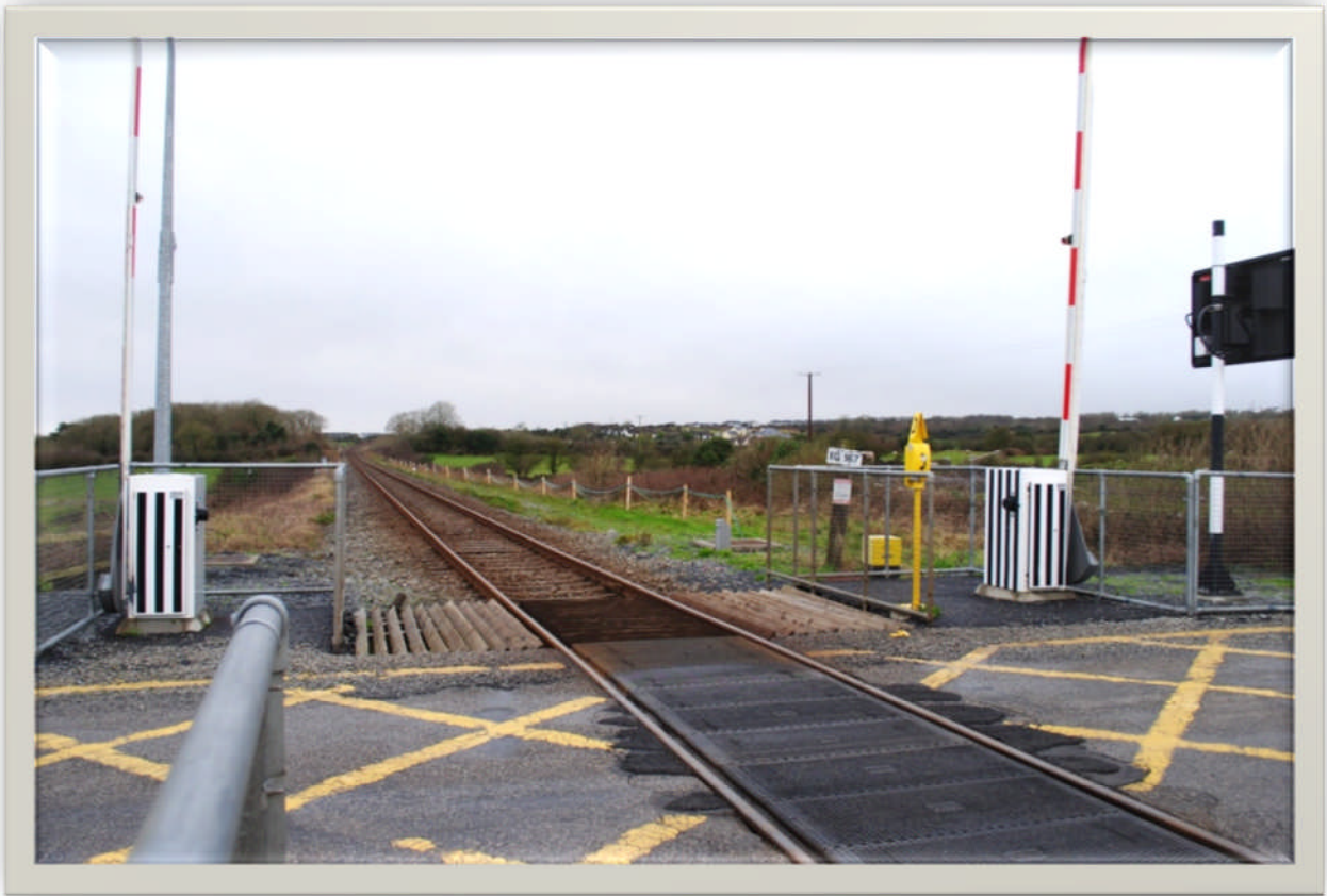
Photo 9. Railway Line at Garraun.
